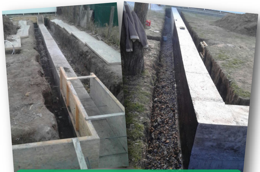
Foundation of the new auditorium. Left picture shows the rear wall and the right picture shows what will be the front of the building.
